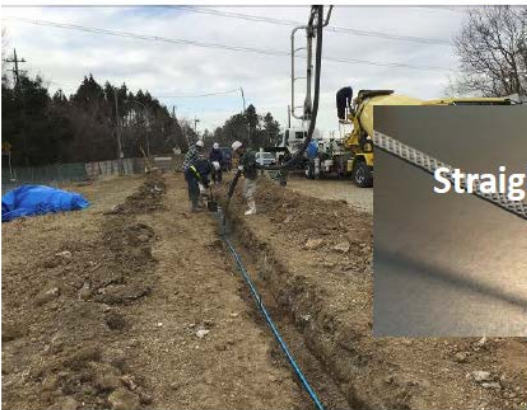
fiber cable covered with Soil (Left) and Cement (Right)
