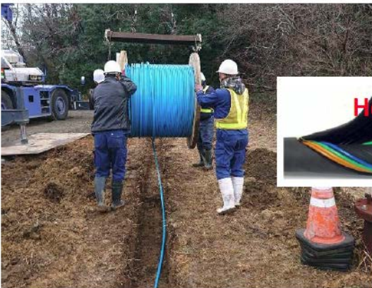
Shallow trench for fiber cable installation
