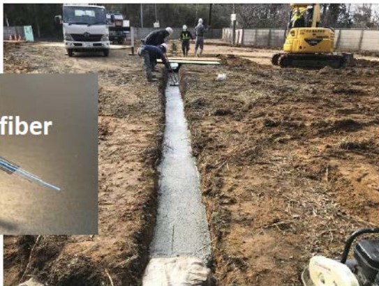
fiber cable covered with Soil (Left) and Cement (Right)
