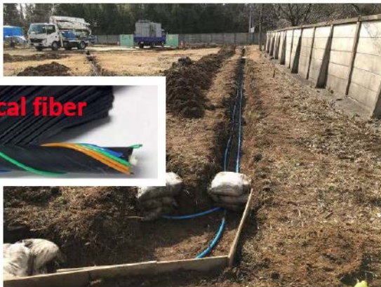
Shallow trench for fiber cable installation
